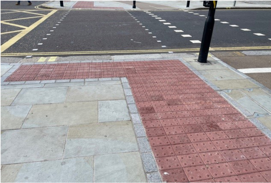
Image 2 - Signalised crossings should be the first type of crossing considered, as they provide certainty for people with sight loss when crossing a road.
