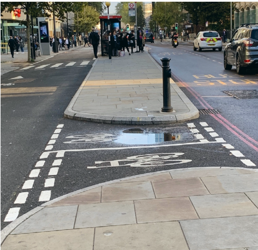
Image 12 - Bicycles are difficult to hear, which makes floating bus stops difficult for people with sight loss to use, as they have to cross a cycle path to reach the bus stop.
