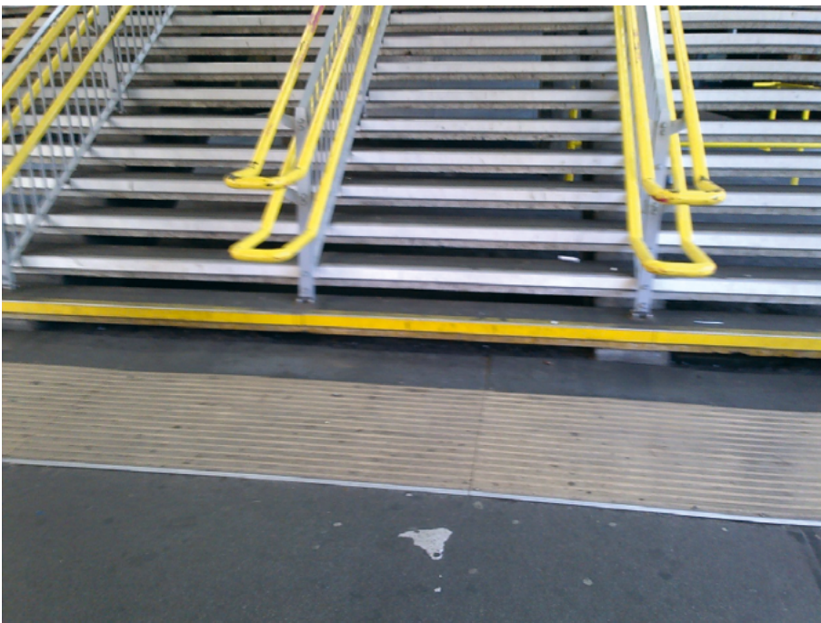
Image 25 - Staircases should have corduroy tactile paving at the top and bottom of stairs. Handrails, the nosings and other features should contrast well against the stairs, so they are easily identifiable.
