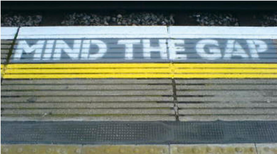
Image 4 - Tactile paving has to be laid in specific places depending on the context. This image shows blister paving laid at the edge of a train platform. There is a yellow warning line running along the edge of the blister paving and another white line 800mm beyond the yellow line on the edge of the platform.
