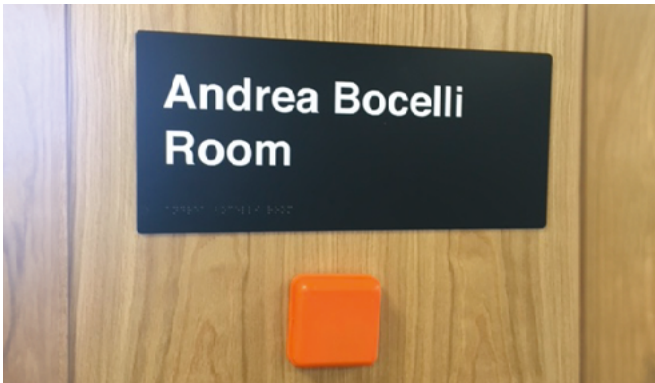
Image 15 – Signage on doors should be: at eye level, have text which contrasts well against its background, contain embossed braille. Small audio boxes can also provide crucial additional information.
