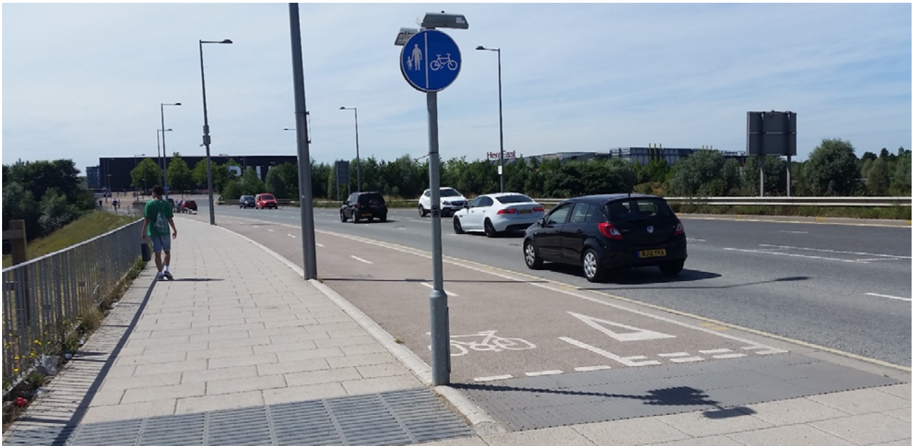
Image 1 - a segregated shared cycle and pedestrian route that conforms to the recommended design guidance.
