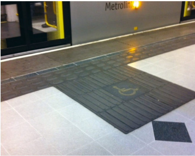
Image 20 - Guidance paving can help identify where the doors of a tram will open.
