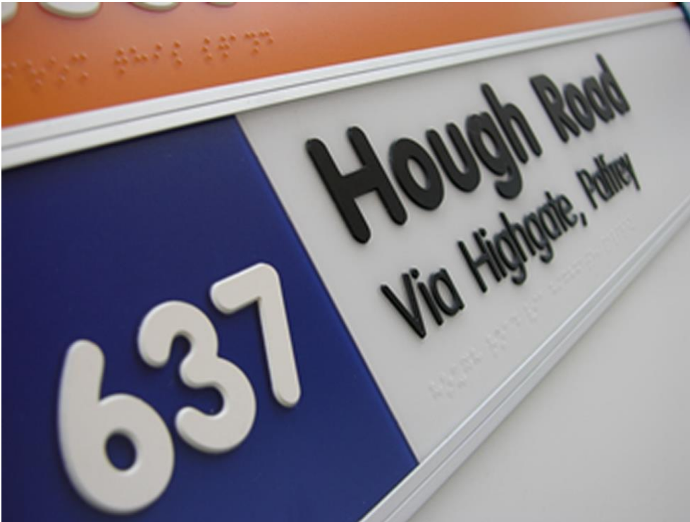
Image 26 – The text on signs in stations and interchanges should contrast against its background. Embossed text and braille should also be used to ensure a sign is accessible.
