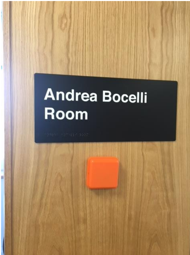
Image 15 – Signage on doors should be: at eye level, have text which contrasts well against its background, contain embossed braille. Small audio boxes can also provide crucial additional information.
