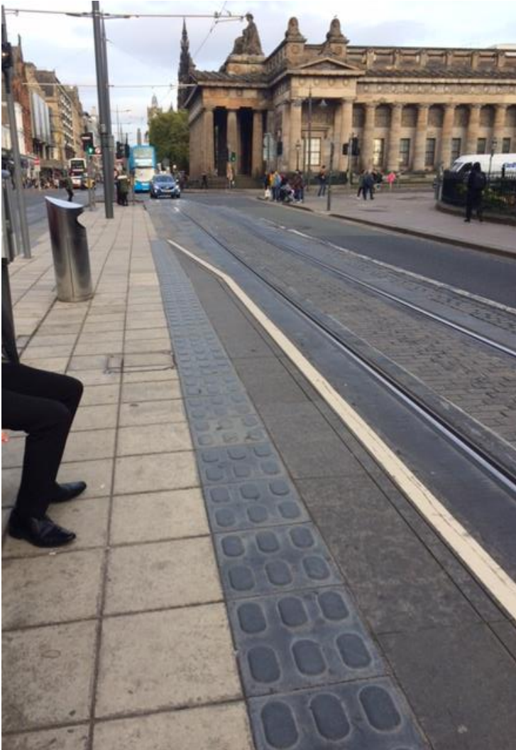
Image 24 - Tram stops should have lozenge tactile paving, approximately 600mm away from the edge of the platform, which should contrast against the rest of the platform.
