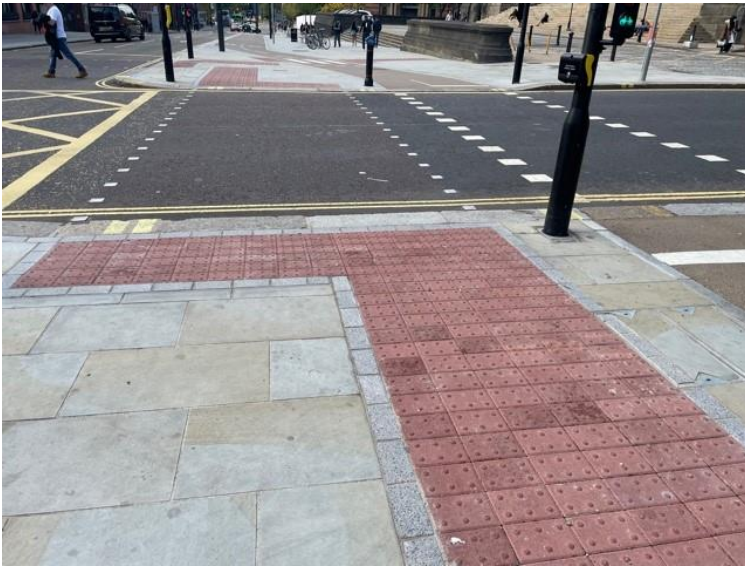
Image 2 - Signalised crossings should be the first type of crossing considered, as they provide certainty for people with sight loss when crossing a road.
