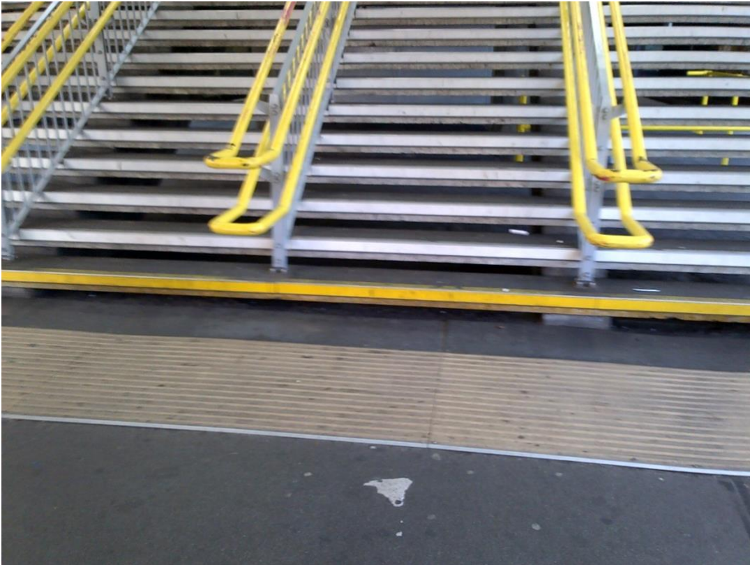
Image 25 - Staircases should have corduroy tactile paving at the top and bottom of stairs. Handrails, the nosings and other features should contrast well against the stairs, so they are easily identifiable.
