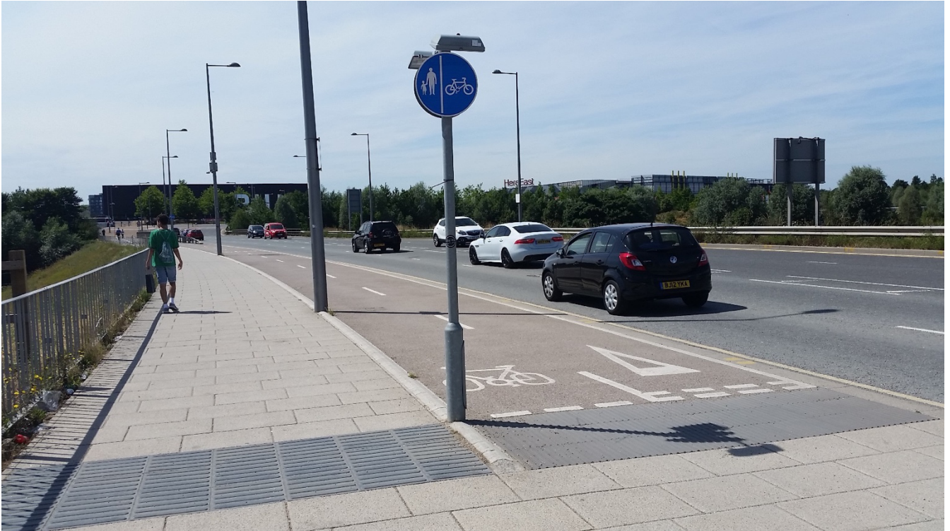
Image 1 - a segregated shared cycle and pedestrian route that conforms to the recommended design guidance.
