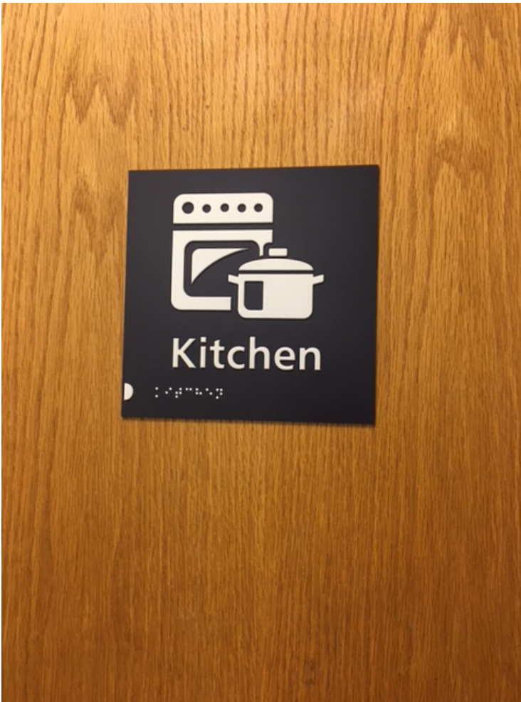
Image 16 - In addition to contrasting text and braille, relevant embossed images can also be used to provide information.
