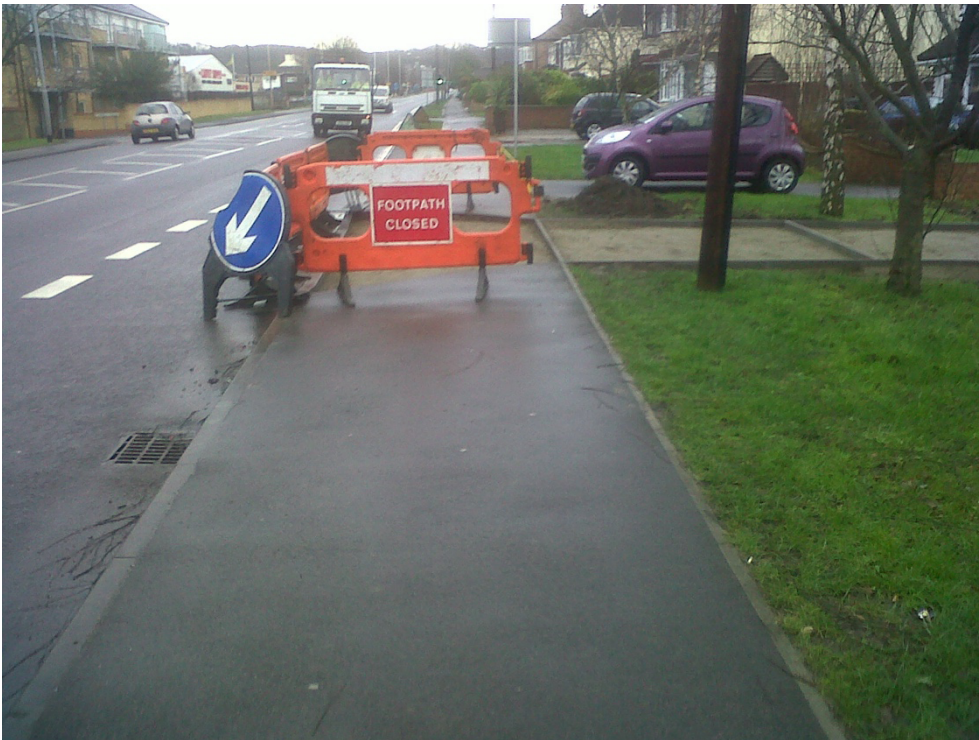
Image 9 - Streetworks can block off pedestrian routes, forcing pedestrians to walk into the road around the barriers.
