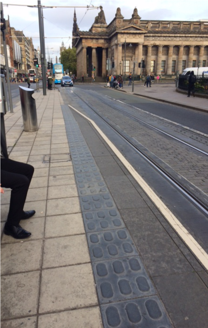
Image 24 - Tram stops should have lozenge tactile paving, approximately 600mm away from the edge of the platform, which should contrast against the rest of the platform.
