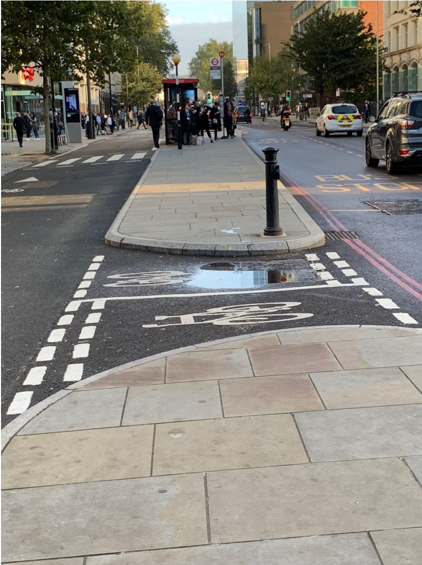
Image 12 - Bicycles are difficult to hear, which makes floating bus stops difficult for people with sight loss to use, as they have to cross a cycle path to reach the bus stop.
