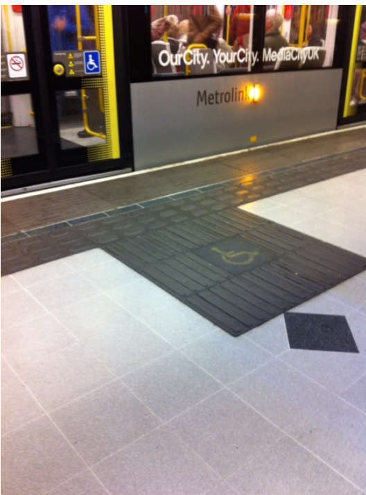
Image 20 – Guidance paving can help identify where the doors of a tram will open.
