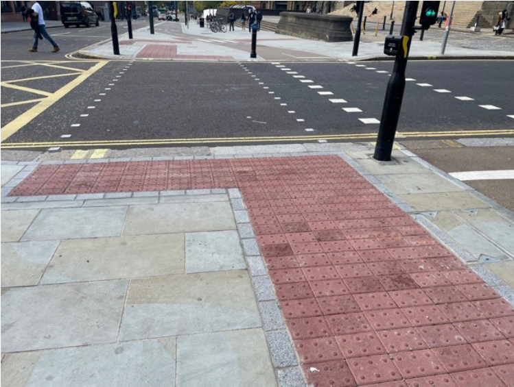
Image 2 - Signalised crossings should be the first type of crossing considered, as they provide certainty for people with sight loss when crossing a road.
