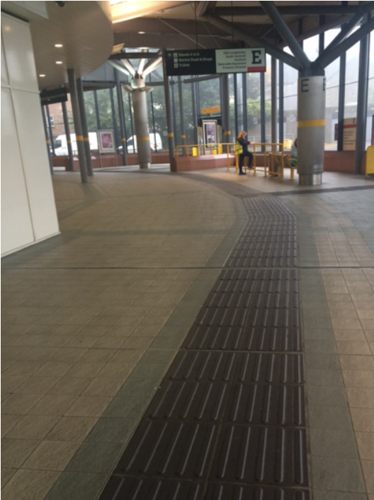
Image 19 – Using tactile guidance paving within stations and interchanges can assist people with sight loss find individual bus bays and other facilities.
