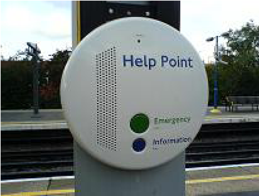
Image 22 - 'Help points' at stations should be easily identifiable, and should have tactile features such as embossed text or braille.
