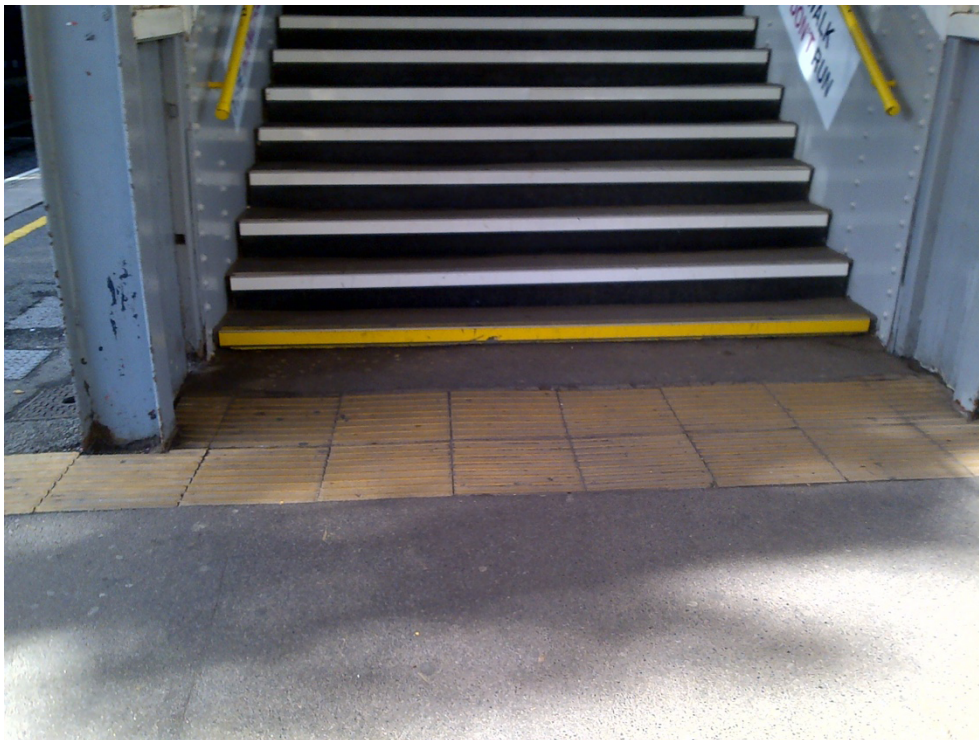
Image 5 - this photo shows ascending stairs with 800mm of buff coloured corduroy paving at the bottom of the last step.
