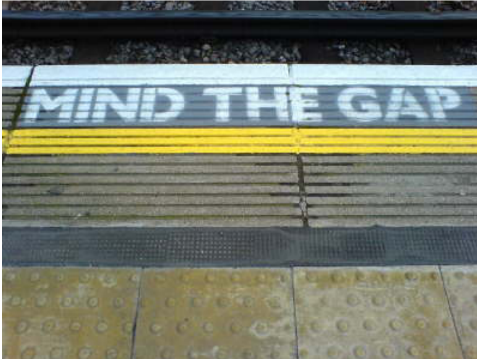
Image 4 - Tactile paving has to be laid in specific places depending on the context. This image shows blister paving laid at the edge of a train platform. There is a yellow warning line running along the edge of the blister paving and another white line 800mm beyond the yellow line on the edge of the platform.
