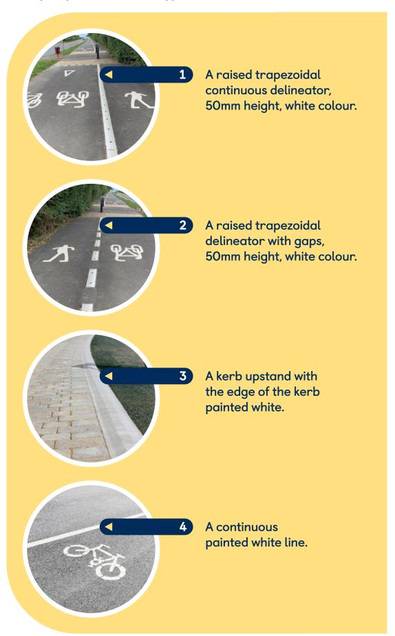
These results found that raised trapezoidal continuous delineators were detected by most users, whereas the raised trapezoidal delineator with gaps was less easily detectable. The kerb upstand was even less easy to detect, and the painted white line came last as the least detectable.
